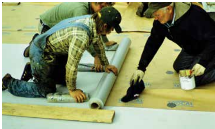
Tetrahydrofuran (THF) was used 35 years ago to chemically weld PVC to a plate-fastened disc. It was "nasty chemically," Dupuis says, and it often caused headaches and dizziness.
