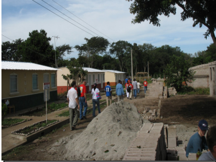
Group worked on houses on right. Houses on left are complete.
