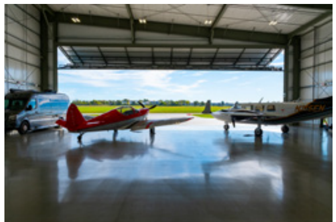
SwiftAir Private Hangar at Wright Brothers Airport LJB Inc.
