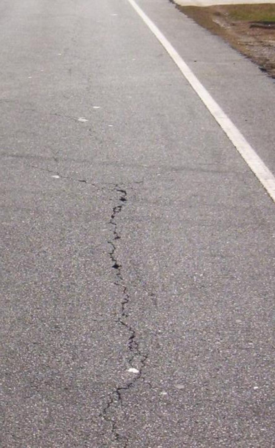
A close-up photograph of asphalt pavement showing a longitudinal crack. The crack runs parallel to a white painted line on the road. The crack is irregular and appears to be a moderate severity.
