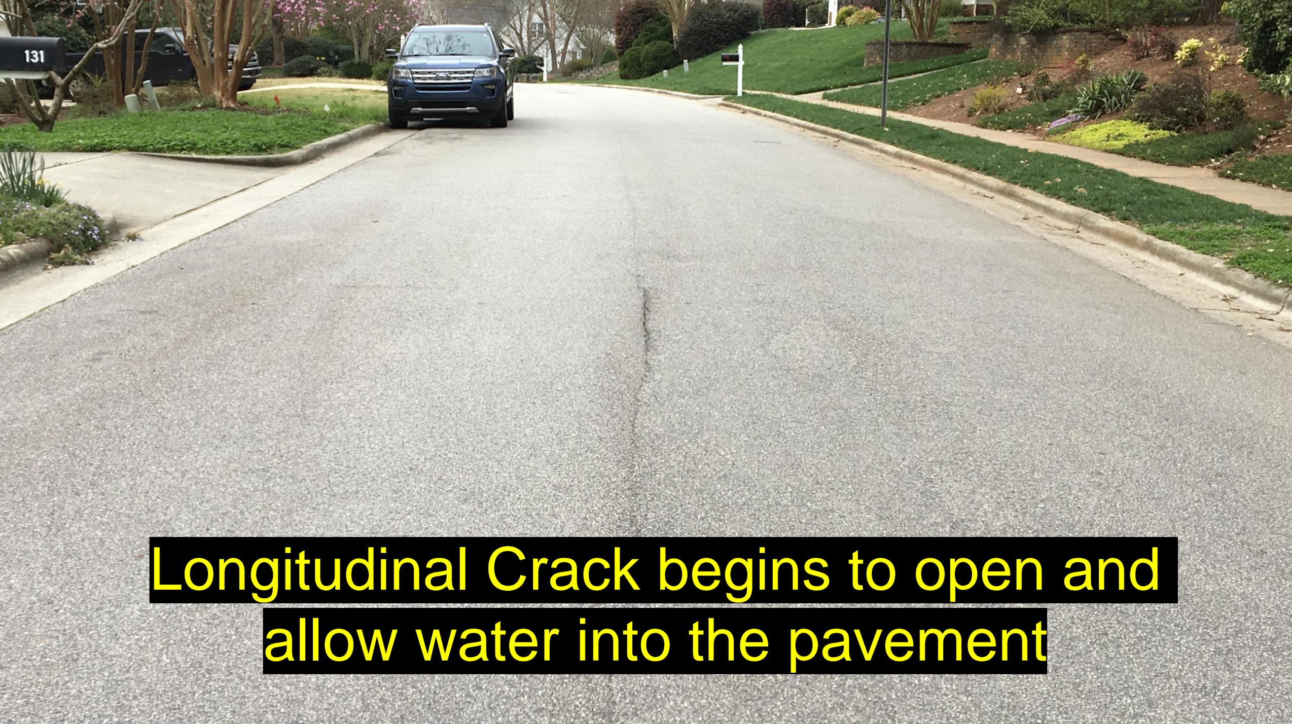
**Longitudinal Crack begins to open and allow water into the pavement**
