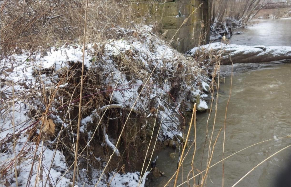
*Figure 9 –Example of a Supplemental Baseline Photo Looking Downstream and Undercut Bank at SE Corner*
