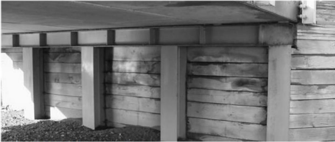
Figure 91 - Steel Capped Bent Abutment with Timber Lagging
