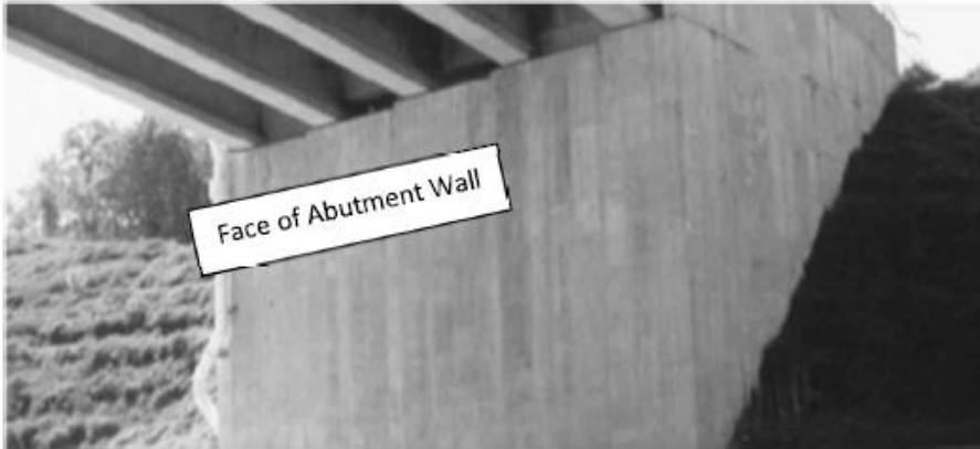
Figure 86 - Full Height Abutment
