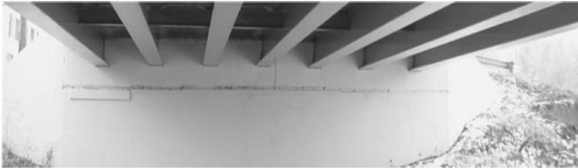
Figure 88 - Semi-Integral Abutment
