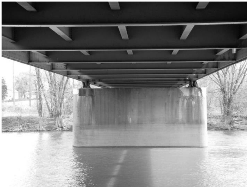
Figure 92 - Pier Wall
