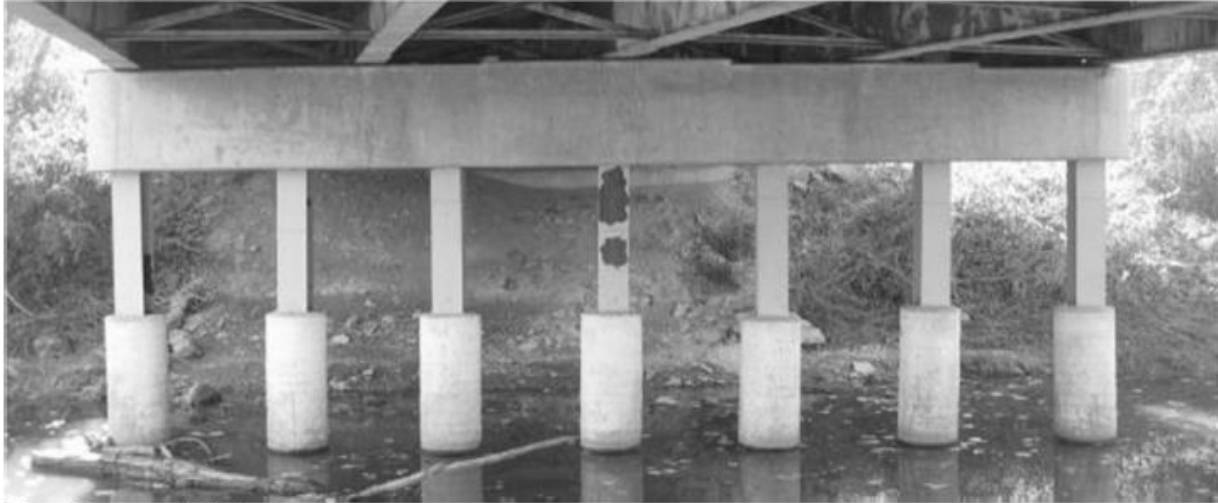
Figure 93 - Capped Bile Bent
