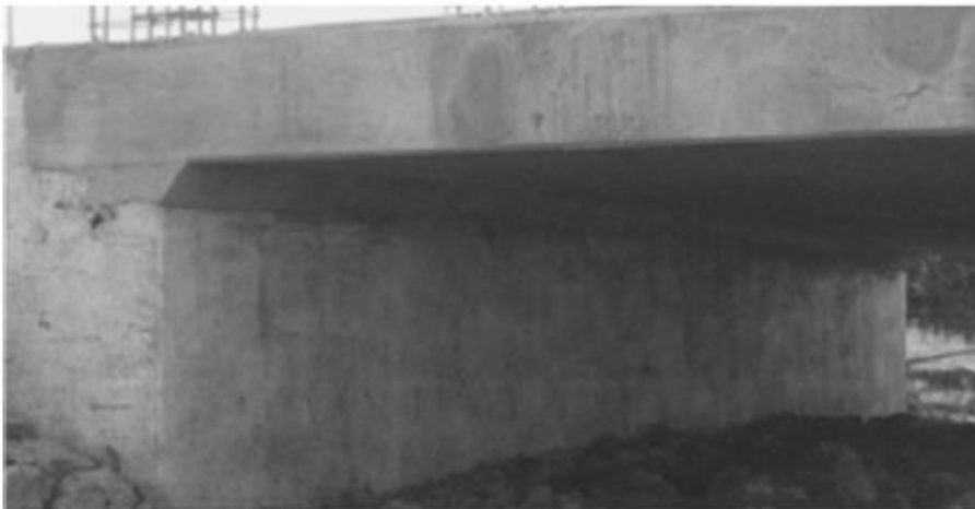
Figure 87 - Stub Abutment
