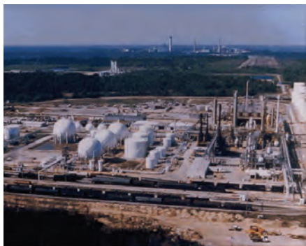
The Plaquemine location comprises three plants—a chlorine and caustic plant, a PVC plant and a VCM plant. This site employs approximately 950 employees and core contractors
