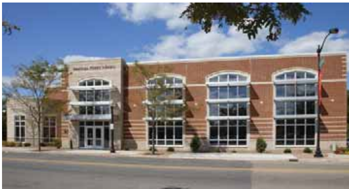
The library’s exterior blends with the 1900s-era façade character of Hastings’s downtown.
