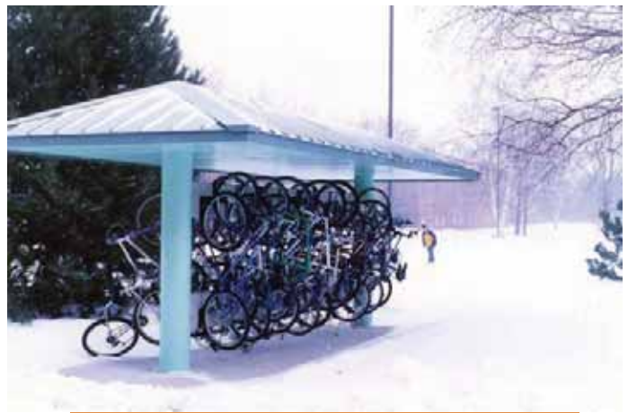
This bike rack at Northern Michigan University was designed for the winter bicyclist and to enable efficient snow clearing operations. Photo by Bill Sanders, UPEA
