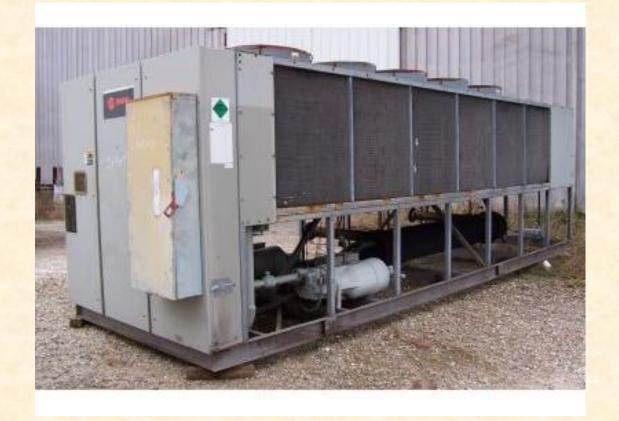
Chillers should be equipped with sound attenuating material and/or baffled with a noise barrier.
