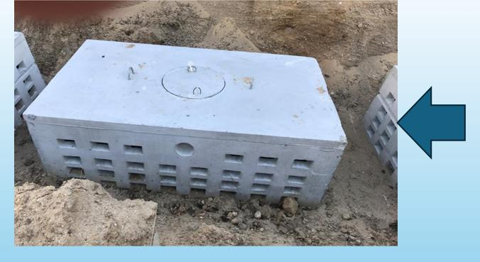
A single leaching galley with 1 ' of aggregate used to simulate the use of a round leach pit ...
