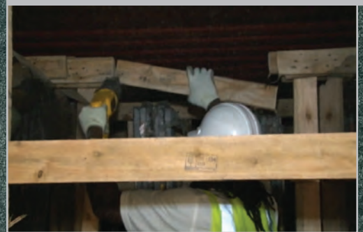
Worker removing braces from a closed-top container
