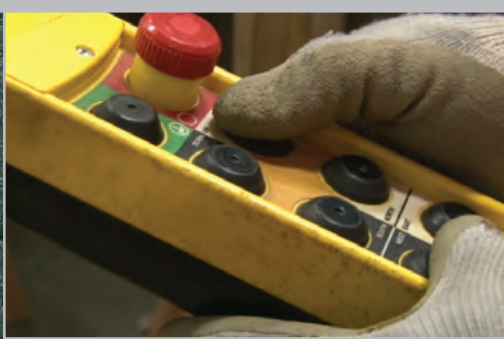
Inspection of hoist controls and brakes
