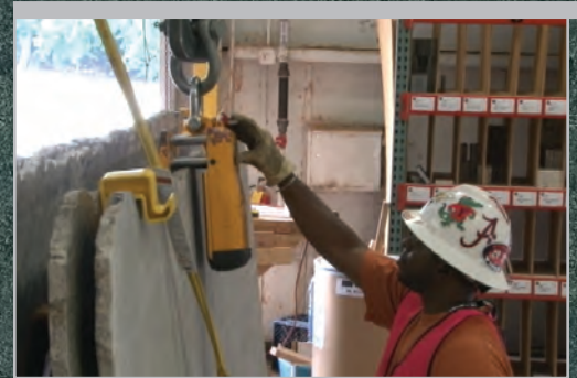
Clamp being properly positioned
