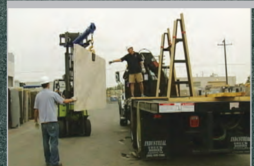
Loading a slab onto a flatbed truck with an A-frame
