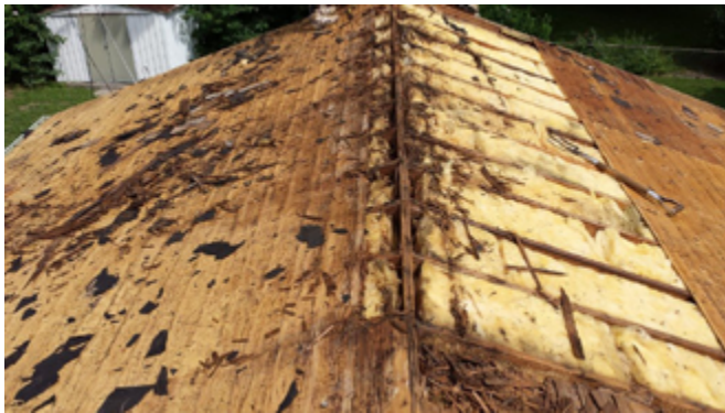
The condition of plywood on a room addition with plenty of attic insulation but zero ventilation; photo courtesy of Epic Exteriors.
