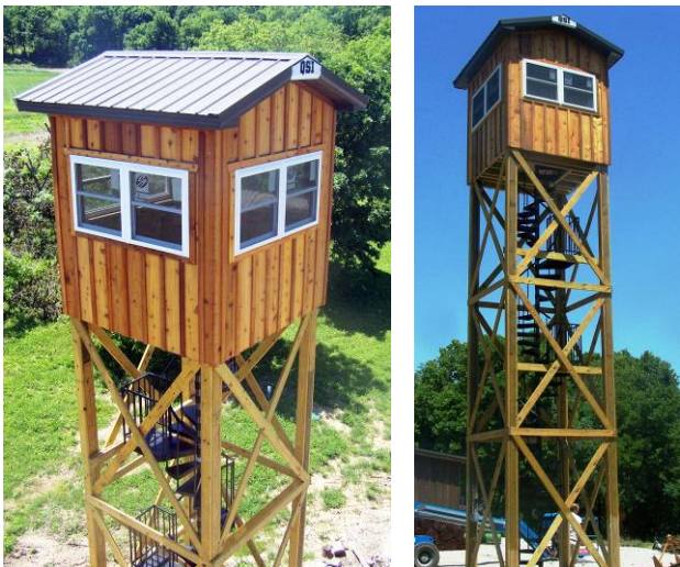
Figure 1-64. Lookout for observing nature, hunting and outdoor recreation. Stands 30 ft. from ground to floor, and 41 ft. to the peak of the roof. The building features 44-ft. long foundation-grade treated four-ply laminated columns on 4 ft. deep embedded footings.
