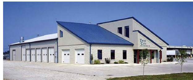
Figure 1-39. Post frame readily accommodates the overhead doors required for this automobile repair business in Lafayette, Indiana. An FBi Buildings project.
