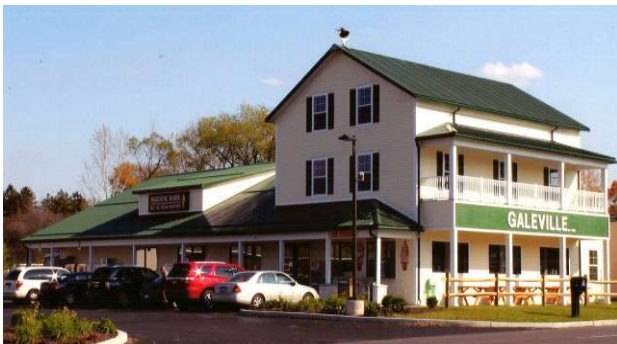
Figure 1-66. Post-frame convenience store for Byrne Dairy in Galeville, NY. The storefront features a porch and above balcony. A porch formed by a roof overhang extends along the side of the structure.
