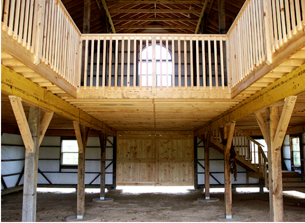
Figure 1-50. Supporting mezzanines with posts instead of walls provide for more open floor plans.
