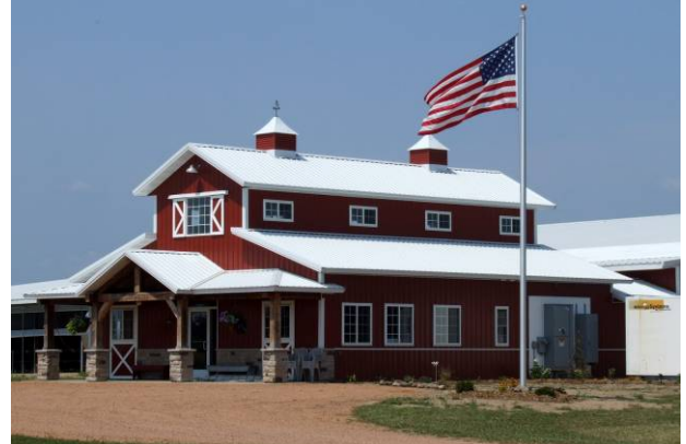
Figure 1-52. Commercial building (top) and milking center (bottom) with clerestories.
