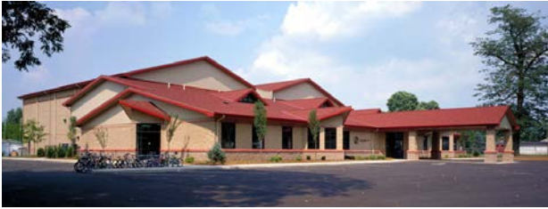
Figure 1-32. Post-frame boys and girls club with steel siding and brick veneer. An FBI Buildings project.
