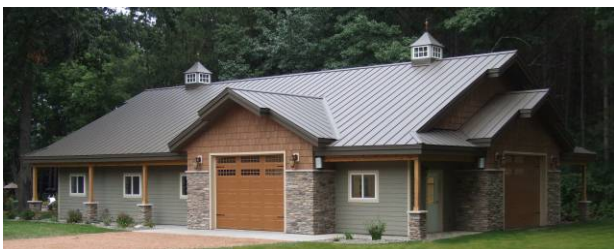
Figure 1-35. Residential post-frame building with brick veneer and fiber-cement board siding.
