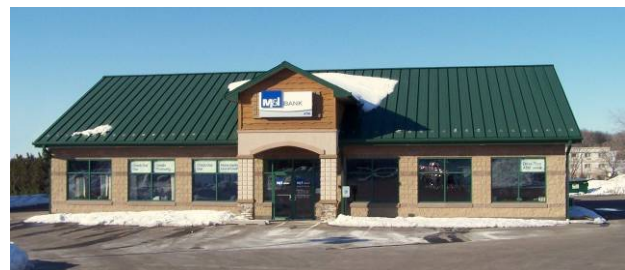
Figure 1-40. Large, equally spaced windows suit post-frame.
