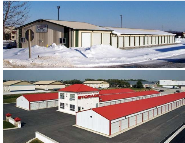
Figure 1-37. The numerous, equally-spaced overhead doors of mini-warehouses make them ideal for post-frame.
