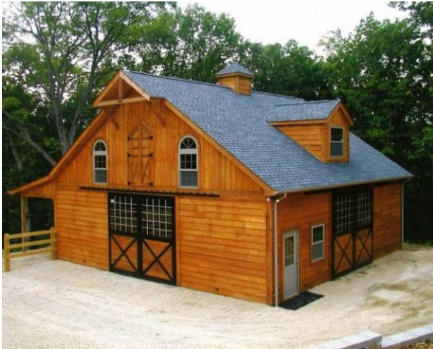
Figure 1-33. Wood-clad post-frame building constructed for horse housing.
