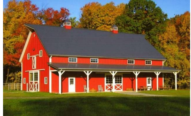
Figure 1-67. Post-frame storage/workshop with side porch.
