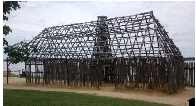
Figure 1-28. Frame of pole building barrack erected in 2011 in an effort to duplicate construction methods used during the colonization of Jamestown. Located behind the replicate barrack is a replicate palisade.
