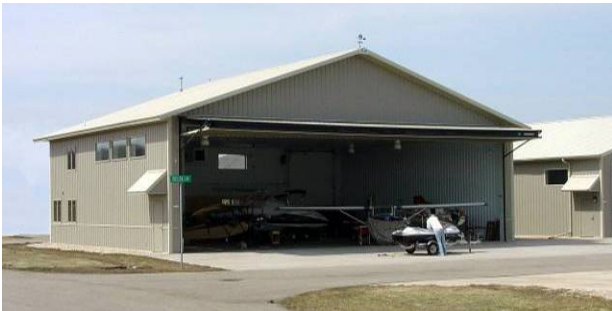
Figure 1-43. The ability to construct inexpensive buildings with relatively high eave heights makes post-frame ideal for many machinery storage buildings including this airplane hanger.
