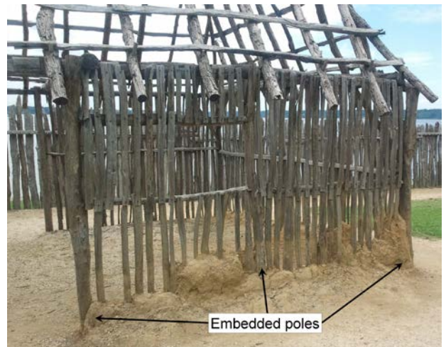
Figure 1-29. Close-up of the barrack shown in figure 1-28. Embedded poles support a girder which in turn supports rafters. Note the similarities between this construction and that shown in figure 1-3.
