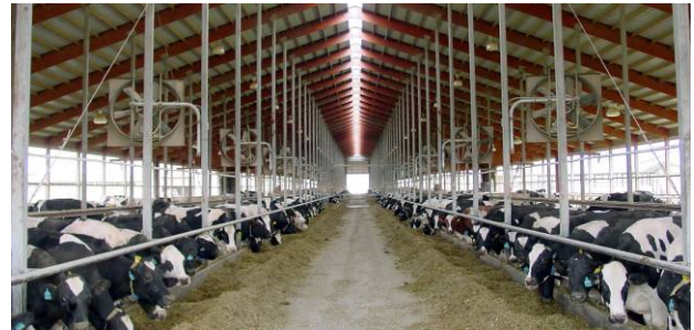
Figure 1-44. This building is typical of many dairy freestall barns. The greater width of these buildings results in (1) tall gable endwalls requiring substantial framing, and (2) the need for interior support posts.
