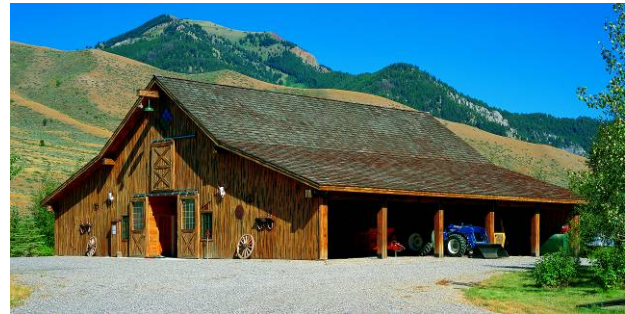
Figure 1-48. Open front equipment storage building.
