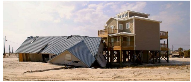
Figure 1-60. Sound engineering and construction of this post-frame stilt building on Dauphin Island, Alabama saved it from meeting the same fate as the one deposited in its front yard by Hurricane Katrina. FEMA photo.
