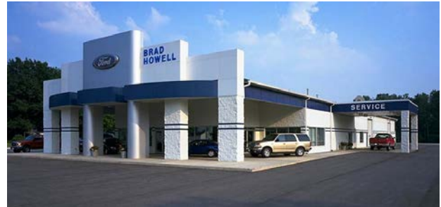
Figure 1-36. Commercial post-frame building clad in stone and smooth metal panels. An FBI Buildings project.
