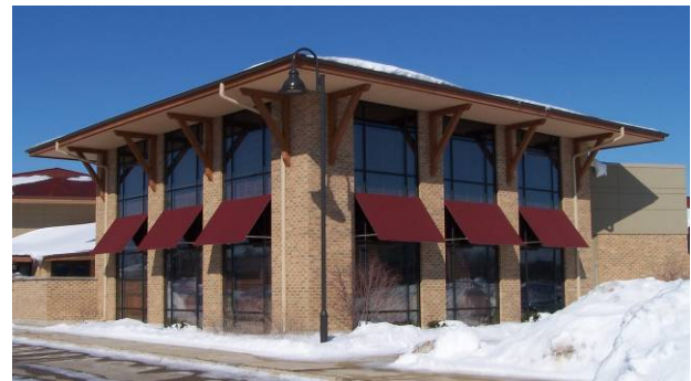
Figure 1-76. Tall walls, large regularly-spaced windows and wall brackets make buildings similar to this good candidates for post-frame.
