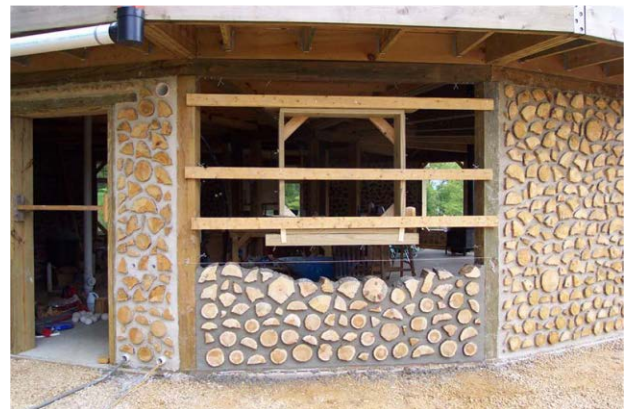
Figure 1-57. Cordwood (a.k.a. stackwood) infill walls.
