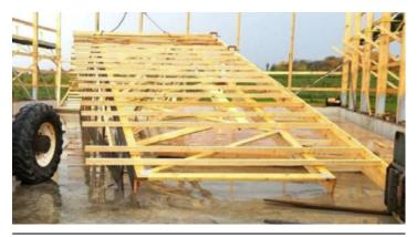
Figure 5. Ground assembly of a bay of roof framing that includes two diaphragm trusses (one on each side of the ridge). possible to the diaphragm truss prior to lifting it in place (figure 6). This approach significantly reduces working at height, and placement of the assembly can generally be managed with a telehandler.
