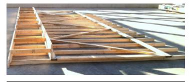
Figure 6. Diaphragm truss with attached purlins and rake overhang framing. Shown in an up-side-down position just prior placement.
