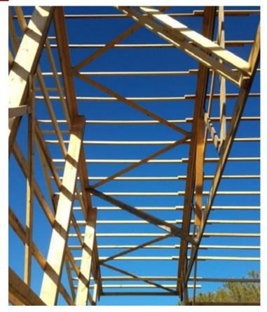
Figure 2. Portion of a diaphragm truss in an end bay
