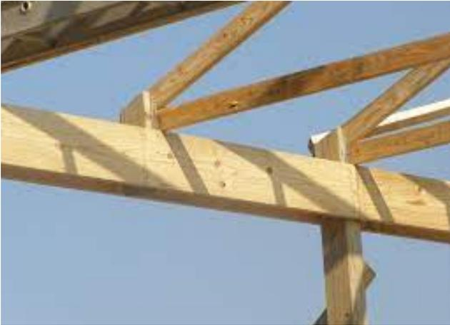
Figure 6 Truss to Column, Truss to Header, and Header to Column Connections: all Critical
