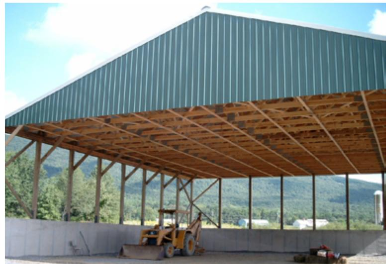
Figure 9 An open-sided building utilizing Knee Braces for Lateral Resistance
