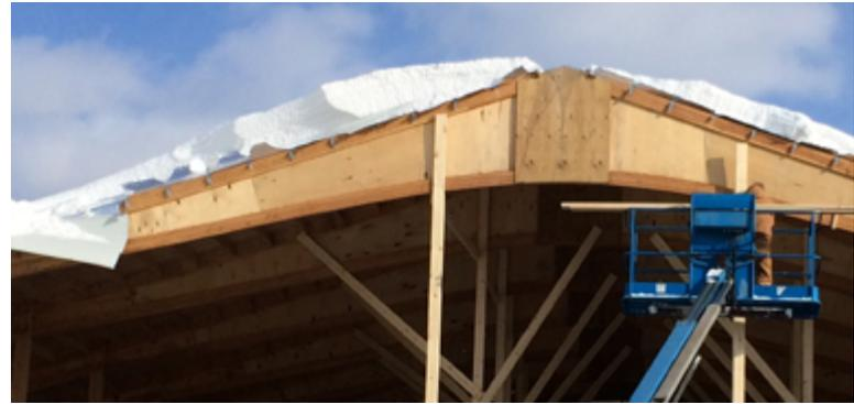
Figure 8 Accumulated Snow drifts at Roof Steps accumulate SIGNIFICANT snow weight on a building
