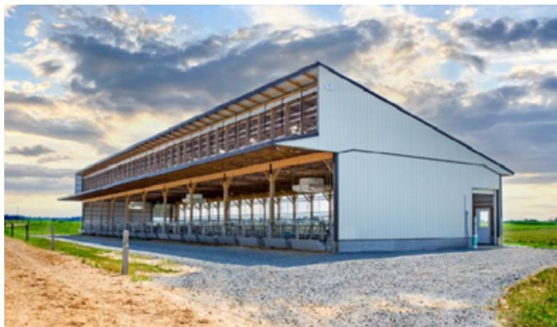
Figure 1 An example of a Partially Enclosed Building
