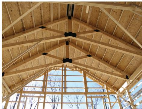
Figure 8. Project 1: Roof framing during construction
