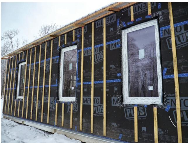
**Figure 16.** Project 3: Exterior view of wall framing and insulation system
