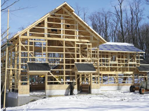
Figure 5. Project 1: Wall framing during construction
