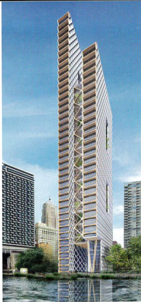
River Beech Tower, another conceptual 80-story mass timber structure, features two side-by-side towers, one slightly taller than the other, above. The facades, below, feature a diamond-shaped diagonal grid system that utilizes laminated veneer lumber elements.
