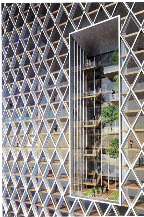
River Beech Tower, another conceptual 80-story mass timber structure, features two side-by-side towers, one slightly taller than the other, above. The facades, below, feature a diamond-shaped diagonal grid system that utilizes laminated veneer lumber elements.
