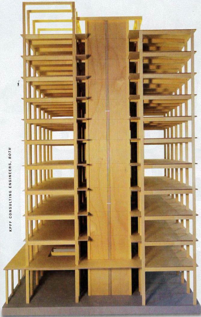
A wooden model, left, assisted in the design of the Framework building in Portland, Oregon. The 12-story, mixed-use building, above, will be the tallest mass timber structure in the United States when completed this year.
