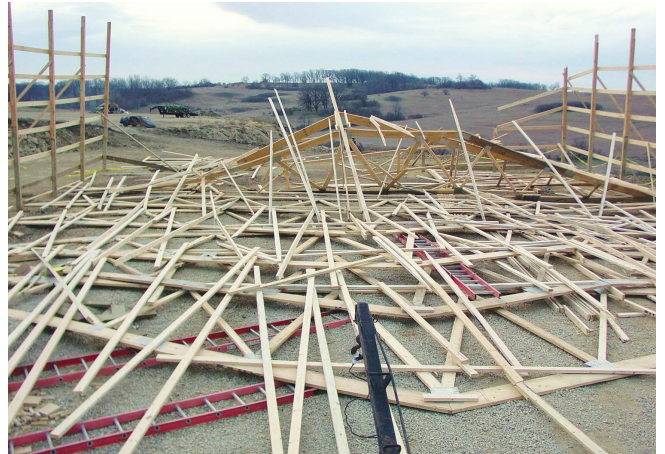
Figure 8. Plan view of roof framing illustrating how a lack of diagonal bracings can result in simultaneous lateral shifting of CLR and truss top chords
