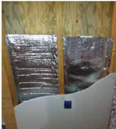
Figure 3. Reflective insulation installed in floor and wall applications
