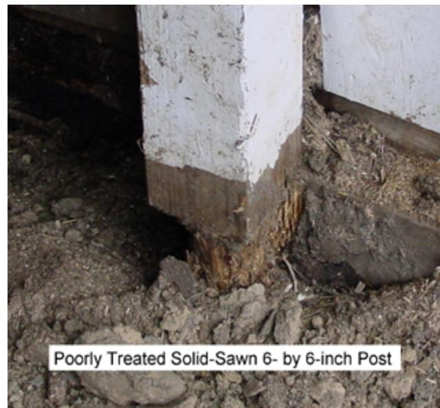
**FIGURE 2. SEVERE WOOD DECAY.**
