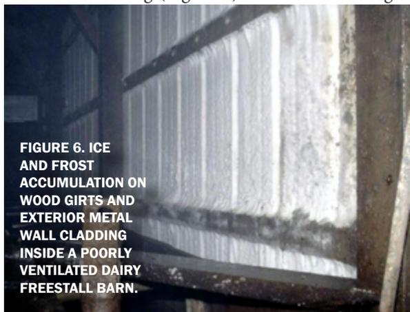
**FIGURE 6. ICE AND FROST ACCUMULATION ON WOOD GIRTS AND EXTERIOR METAL WALL CLADDING INSIDE A POORLY VENTILATED DAIRY FREESTALL BARN.**
