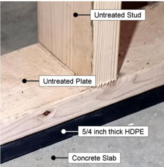
**FIGURE 3. ISOLATING WOOD COMPONENTS FROM A CONCRETE FLOOR WITH HDPE COMPONENTS TO LIMIT WOOD DECAY IN A FOOD PROCESSING FACILITY.**
