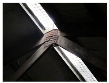
FIGURE 10. CORRODED METAL TRUSS PLATE UNDER AN OPEN RIDGE IN A DAIRY FREESTALL BARN.
