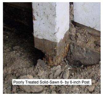
FIGURE 2. SEVERE WOOD DECAY.
