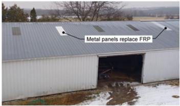
FIGURE 1. REPLACEMENT OF DETERIORATED FRP PANELS WITH WHITE CORRUGATED STEEL PANELS.
