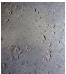
(i.e., excessively power-floated and powertroweled) which removed surface air entrainment.
