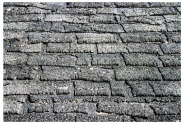
FIGURE 9. BADLY DETERIORATED BLACK ASPHALT SHINGLE ROOF AFTER ONLY 20 YEARS OF SERVICE.
