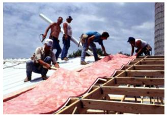
FIGURE 7. INSTALLATION OF VINYL-FACED FIBERGLASS INSULATION BETWEEN WOOD FRAMING AND CORRUGATED METAL ROOFING.
