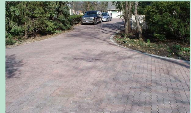
Porous Pavements are increasingly in demand as tools for managing storm water in an environmentally friendly way. They are an alternative to costly, bulky and land-intensive detention or retention ponds.
