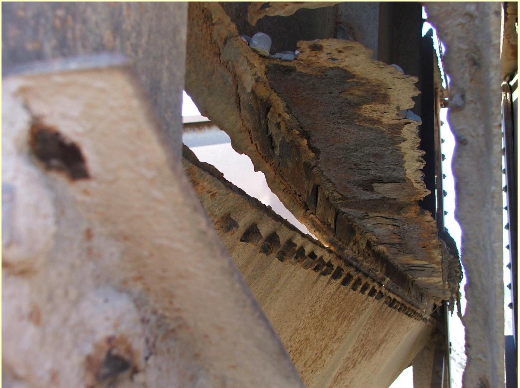
Hopper separation from the bin wall. 62
