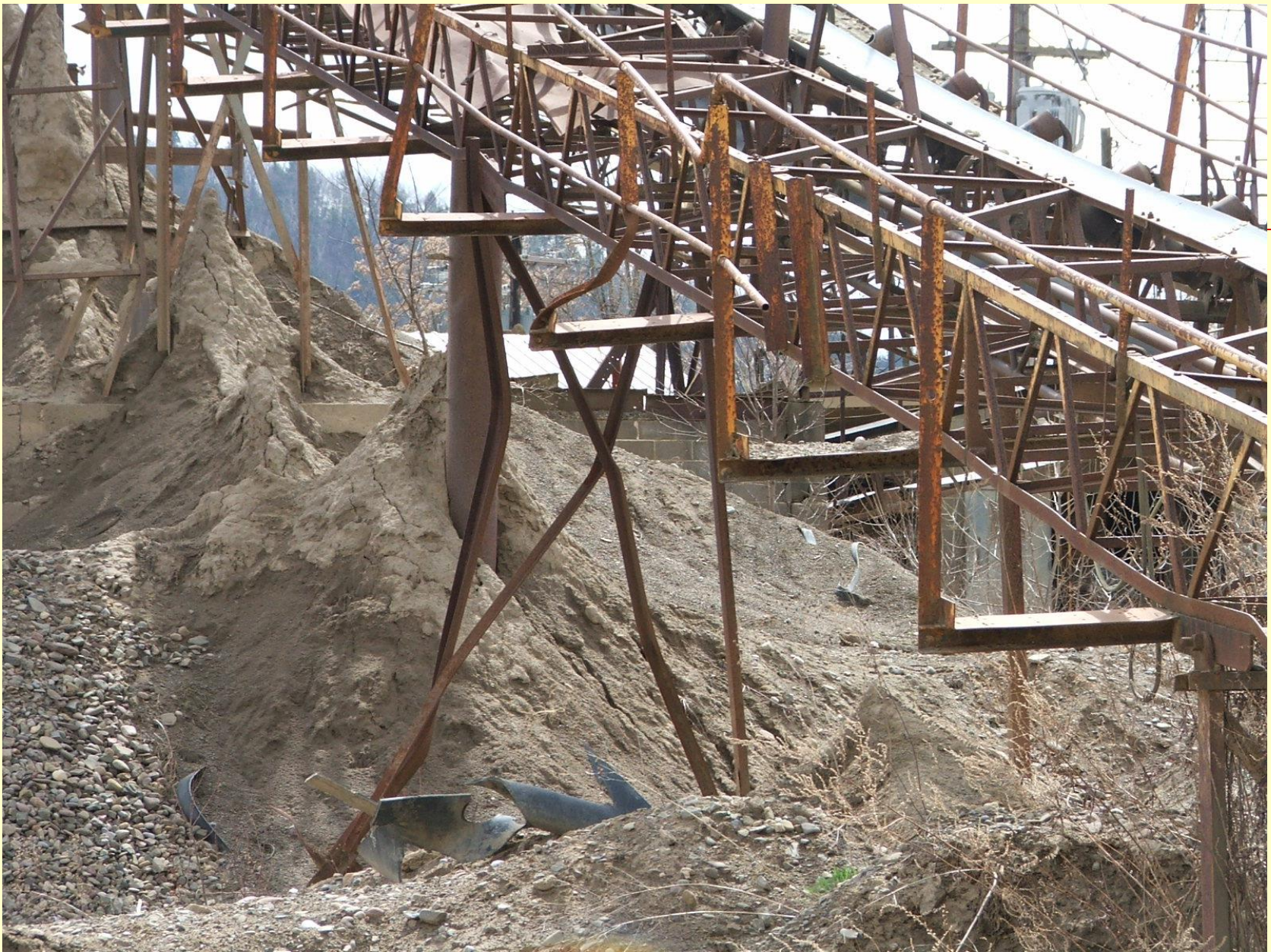
Impact damage to a conveyor bent and excessive material build up
