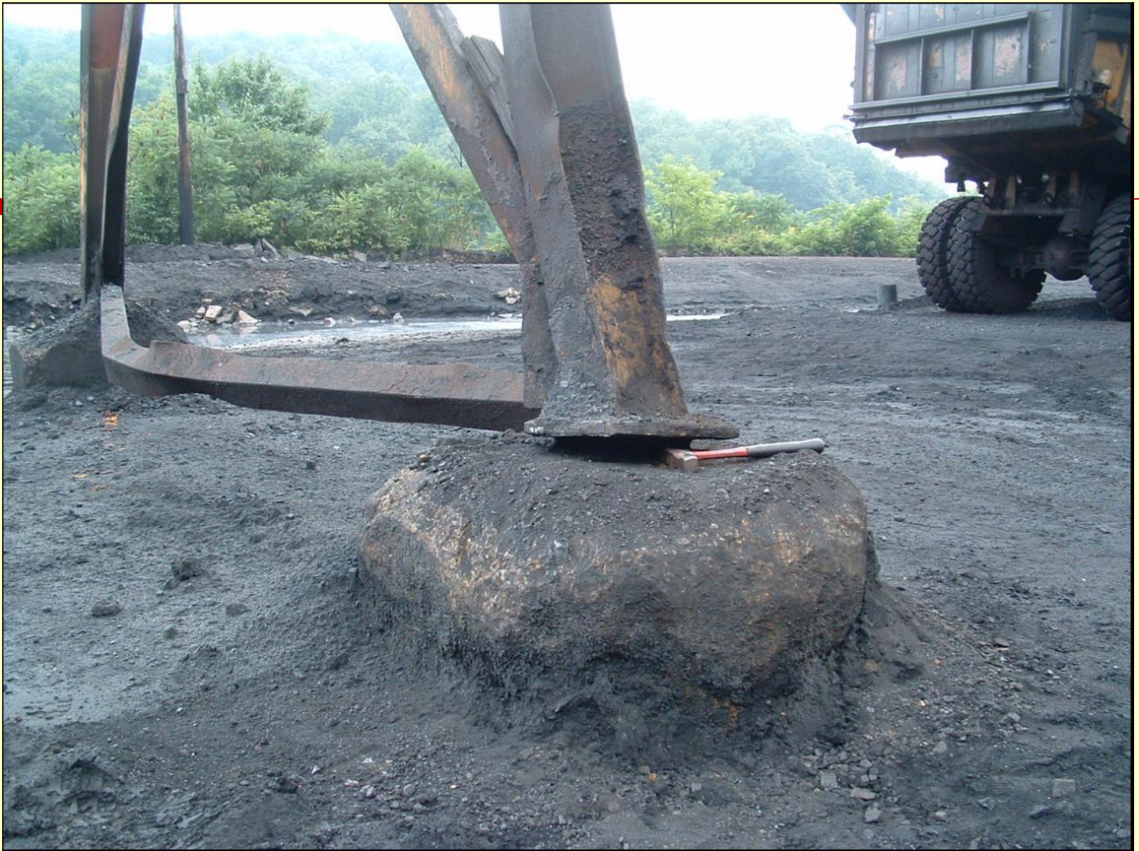
Impact damage - conveyor bent separated from the concrete foundation
