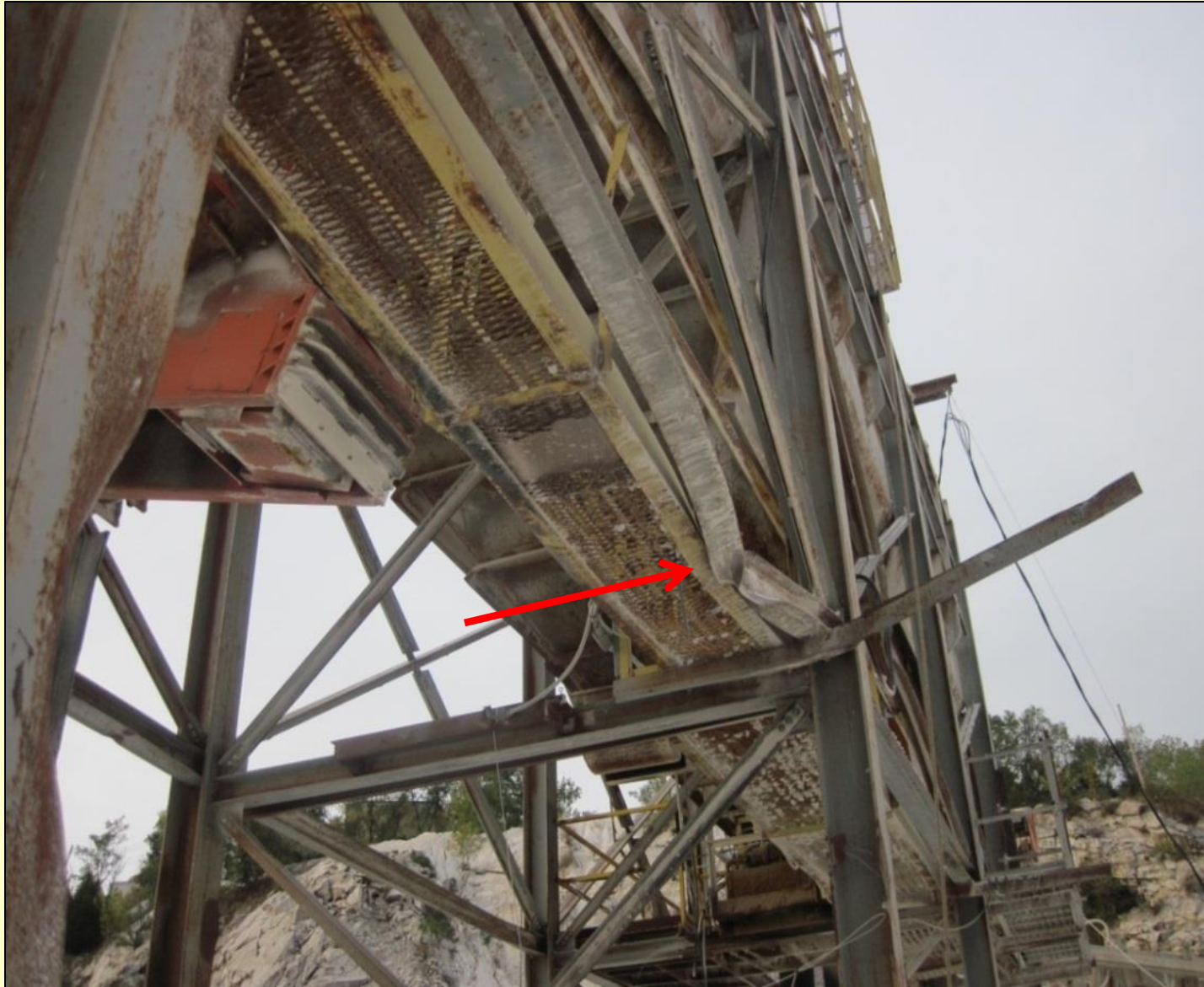
Damaged lateral beam supporting a bin column.
