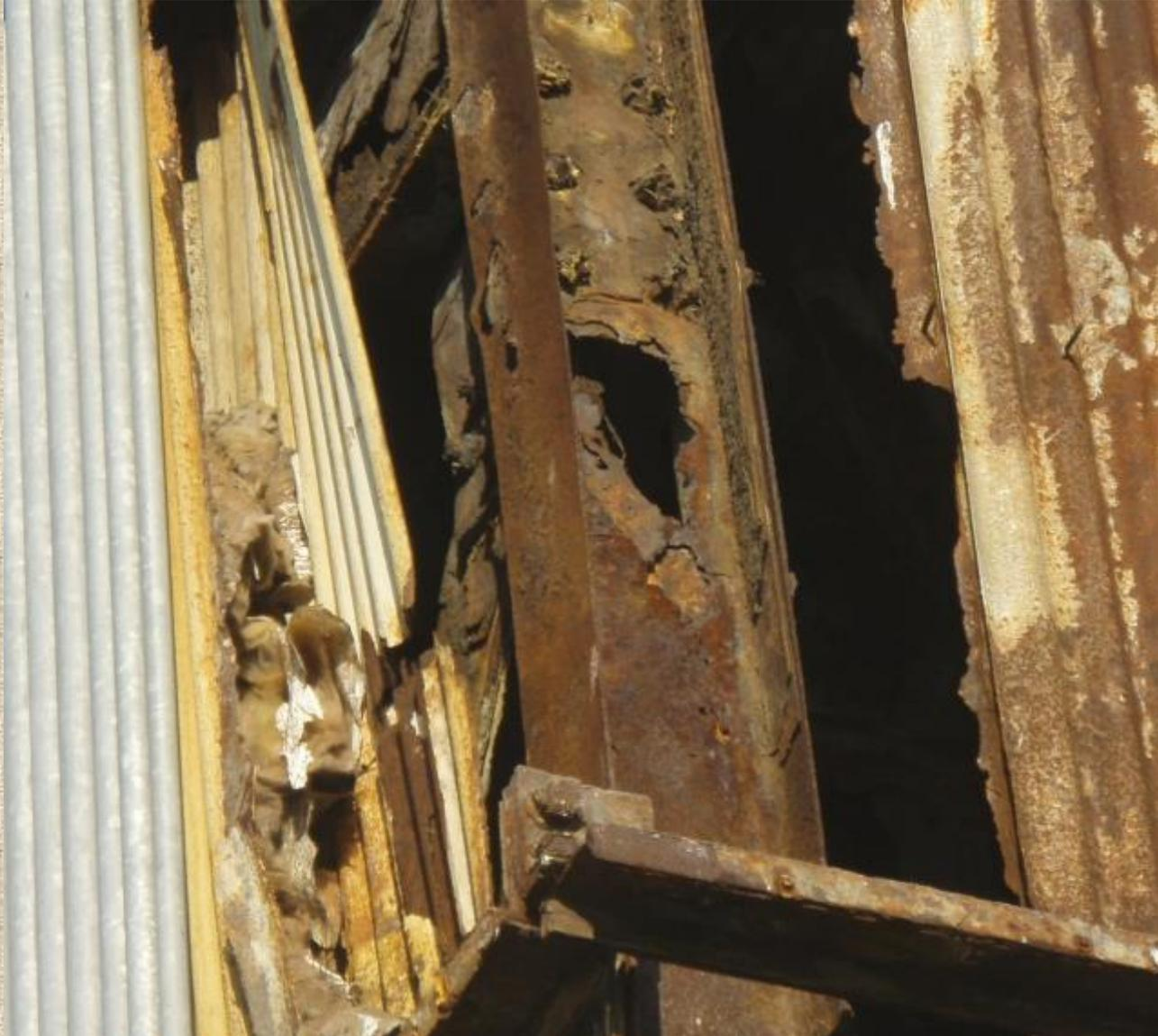
Corroded diagonal braces (and sometimes intentionally removed braces to accommodate equipment changes or access) should be repaired or replaced. Braces are necessary to resist lateral loads such as wind, earthquake, and vibration.
