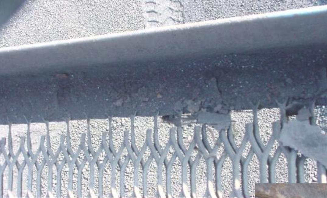
Corrosion at support edge of walkway grating, corrosion holes in a stairway channel stringer, and holes in an angle supporting a tread.
