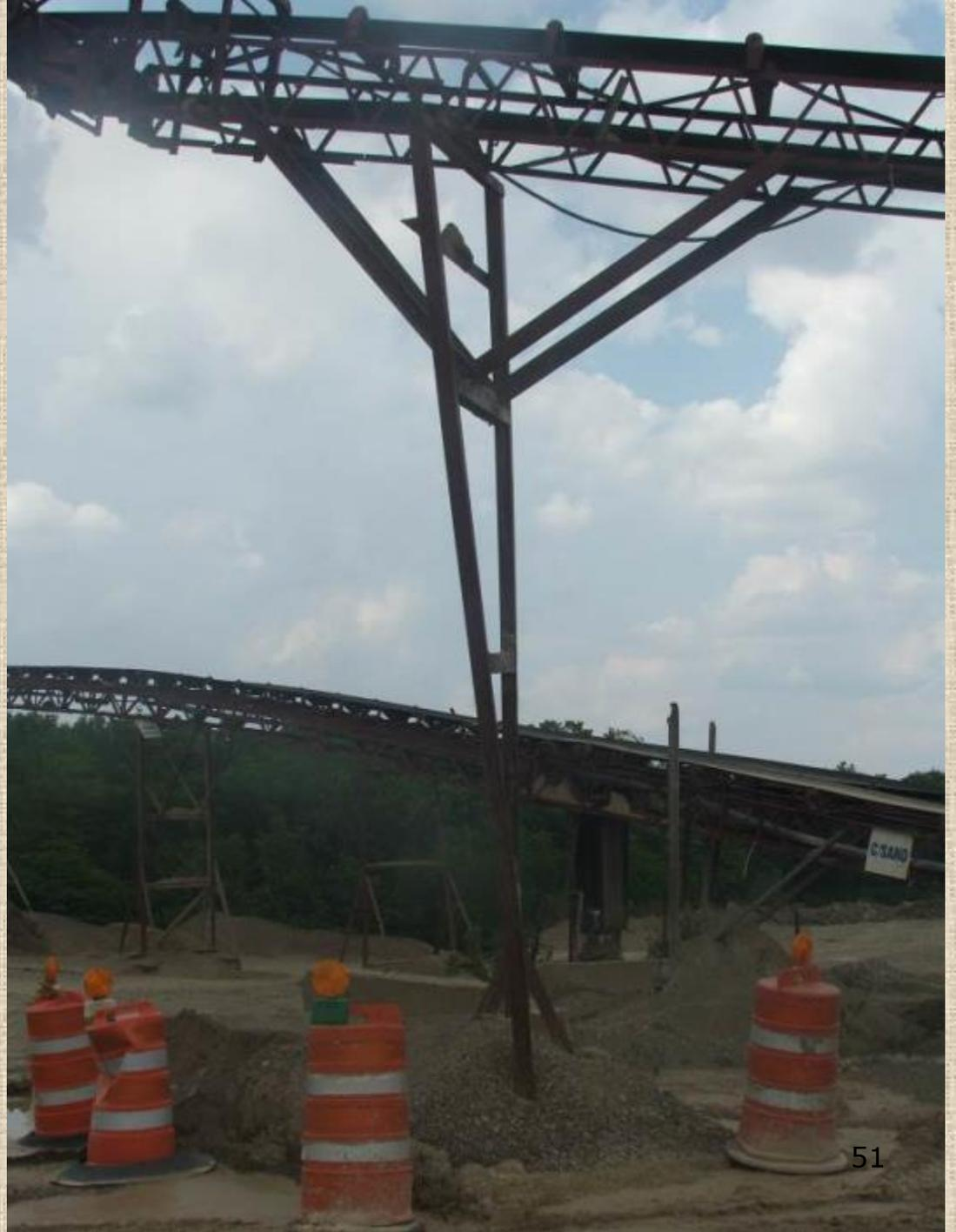
Corroded column at the base of a conveyor support bent.
