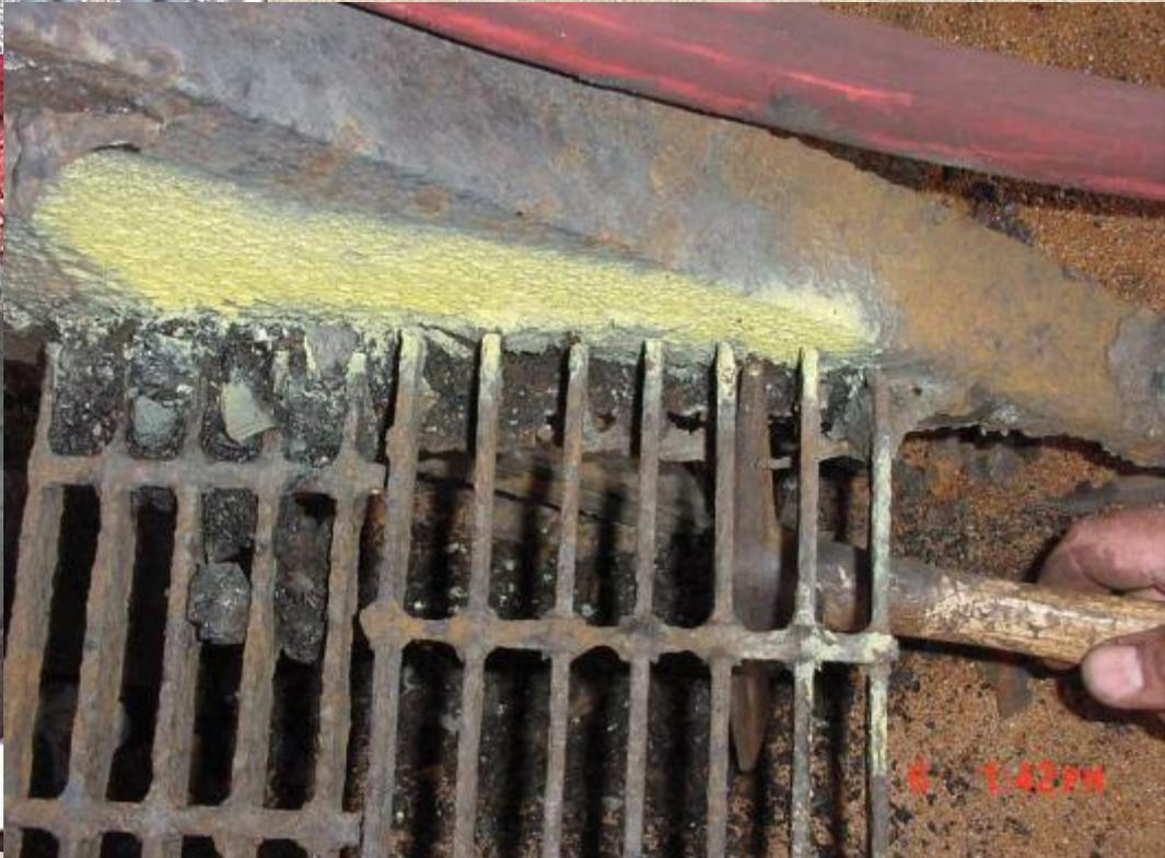
A miner was seriously injured at a limestone mine when the expanded metal walkway suddenly failed. He fell 10 feet to the ground. The expanded metal walkway was covered with conveyor belt to aid in shoveling spillage. The belting allowed corrosive material to accumulate and accelerated the deterioration of the expanded metal. Also the belting masked the signs of deterioration making examination difficult.
