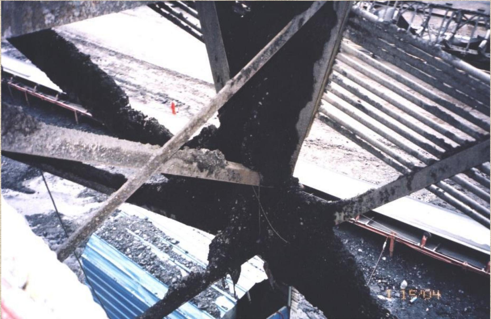
Accumulations on bottom chords and verticals add weight and may<sup>38</sup> facilitate corrosion
