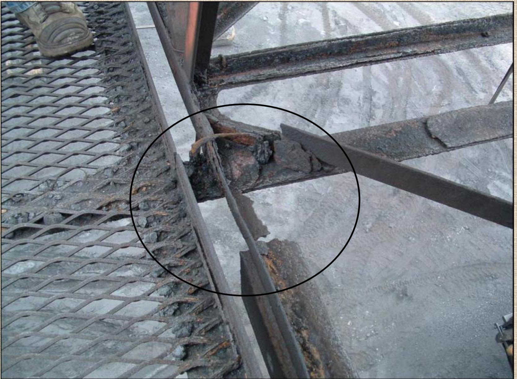
One leg of bottom chord angle corroded through and U-bolt walkway support was also severely corroded
