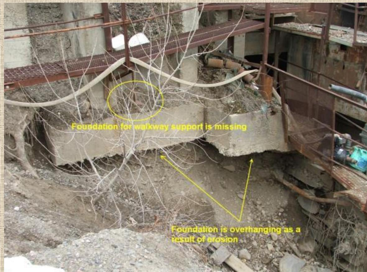
Foundation for walkway support is missing
