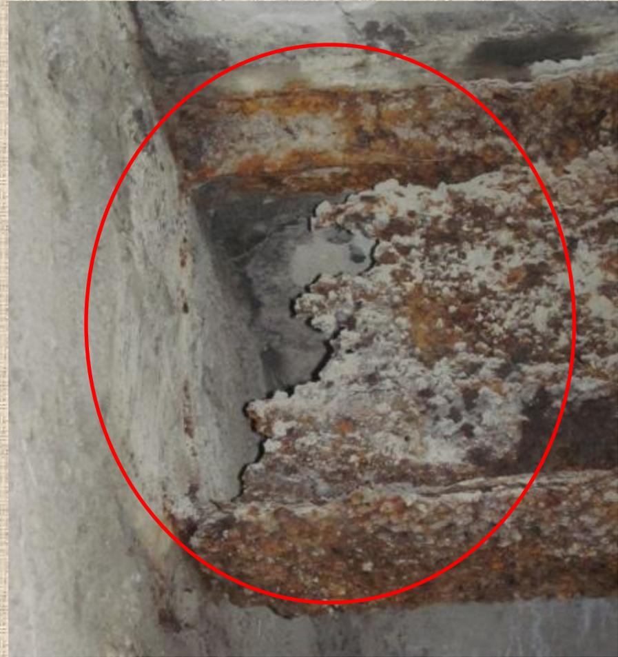
Corrosion holes resulted in web collapse of the back beam.
