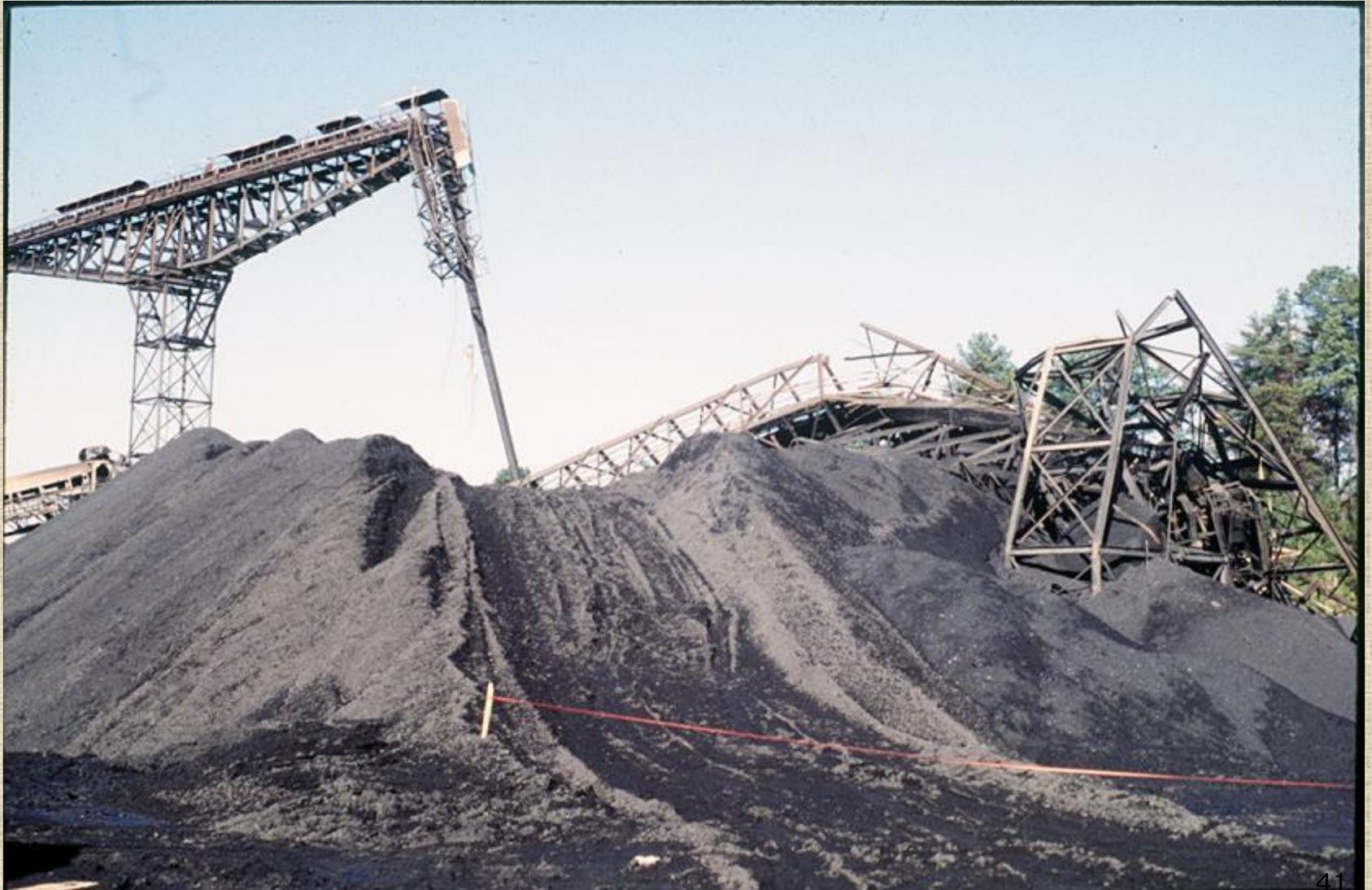
Fractured bottom chord angle section on the truss had 70% loss of cross-sectional area from corrosion.
