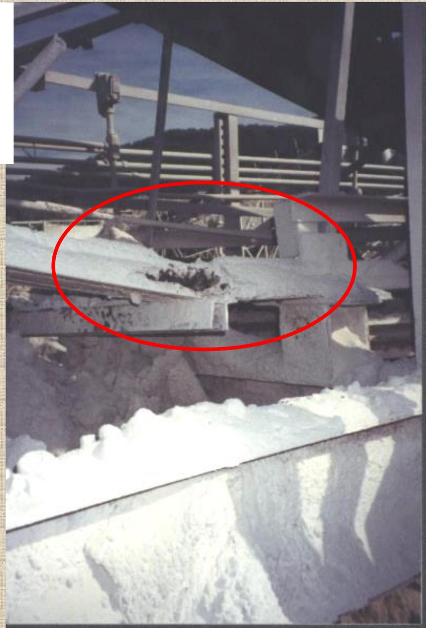
Deflected bottom chord that occurred because an added support post was not located at a joint
