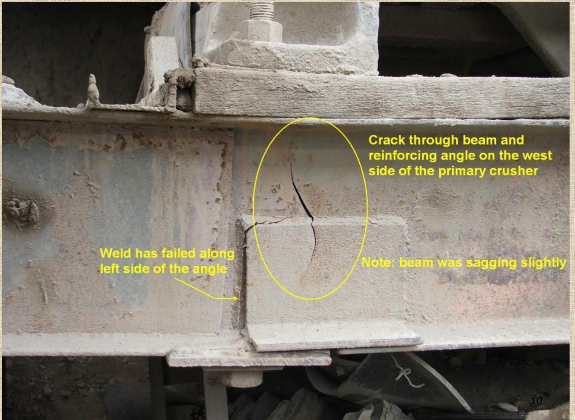
Crack through beam and reinforcing angle on the west side of the primary crusher
