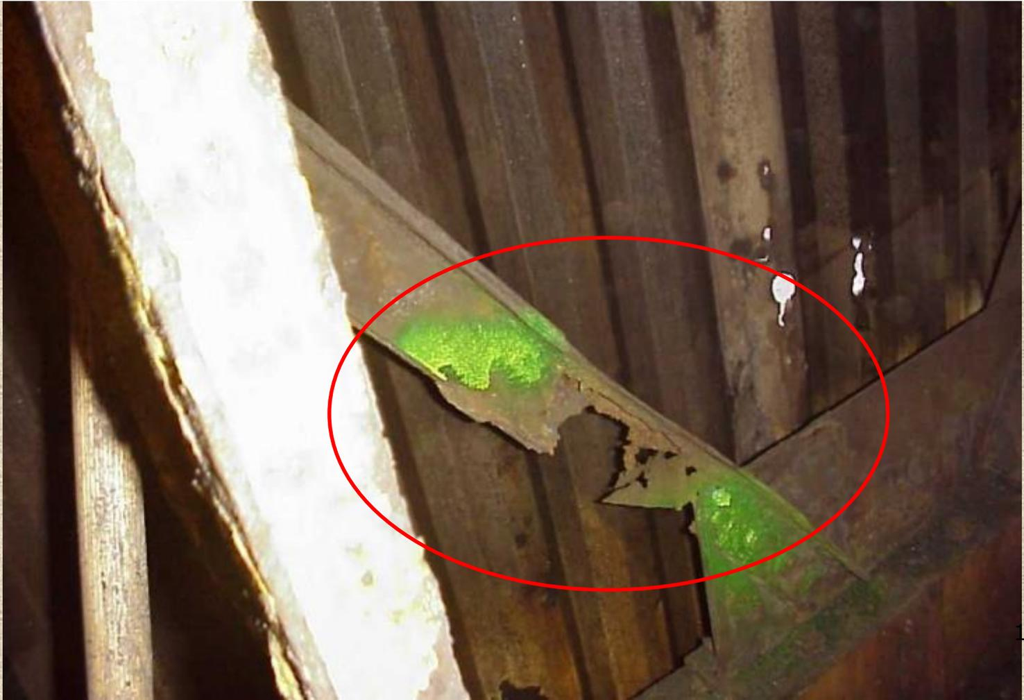
Lines of 100% corrosion along the edges of a floor plate
