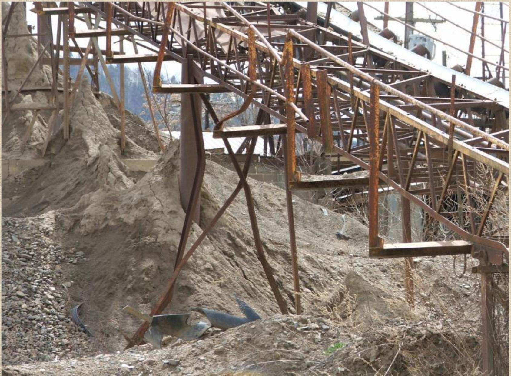
Impact damage to a conveyor bent and excessive material build<sub>up</sub>
