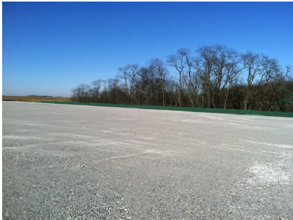
Completed well pad prior to mobilizing the drill rig, December 11th, 2011
