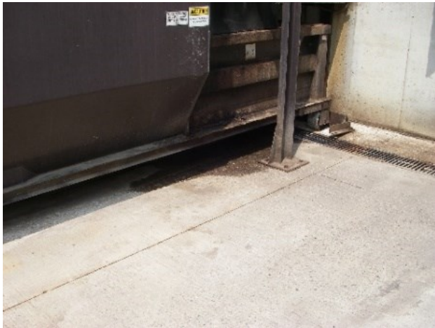
Figure 4: Cleaned up dumpster area (August, 2014)
