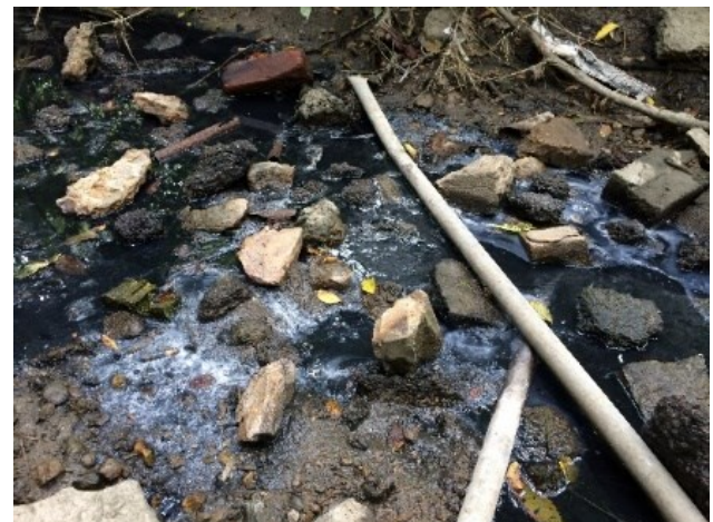
Figure 2: Contaminated water at outfall (August, 2014)
