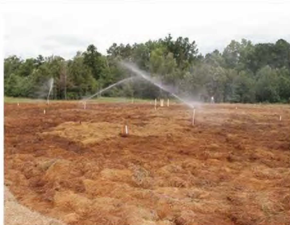
Irrigation system at work –treated site covered in hay
