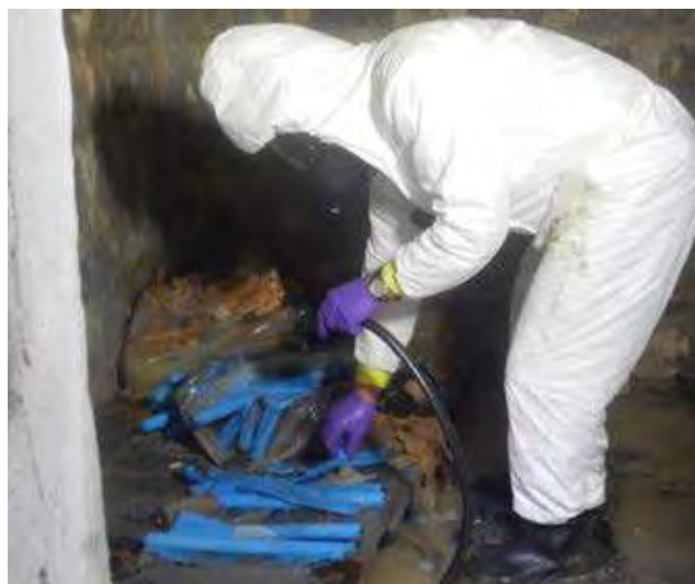
MuniRem UXO technician sprays MuniRem Solution on aged dynamite, weeping Nitroglycerin to render it safe to handle.
