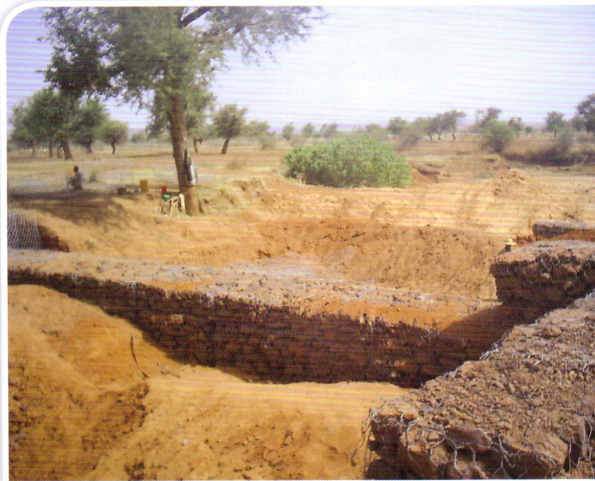
▲ Farmers lay stones in a subsurface dam, which will collect and hold water from underground streams.
